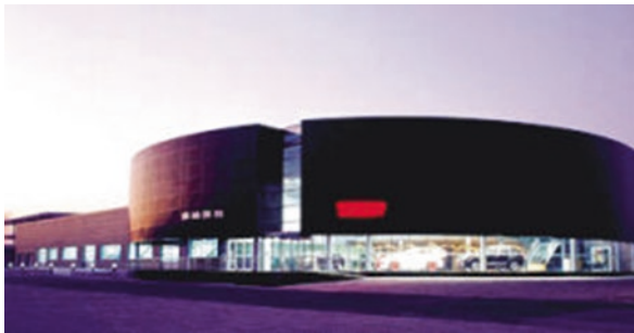
Fig. 1.16 Defendant’s “Taihe Astra Center” (Source: PEI, XIAOLAN. Car modification shop too much alike Porsche building was sentenced to rebuild [N]. Beijing Times, http://news.qq.com/a/20071220/001573.htm , 2007–12–20)
